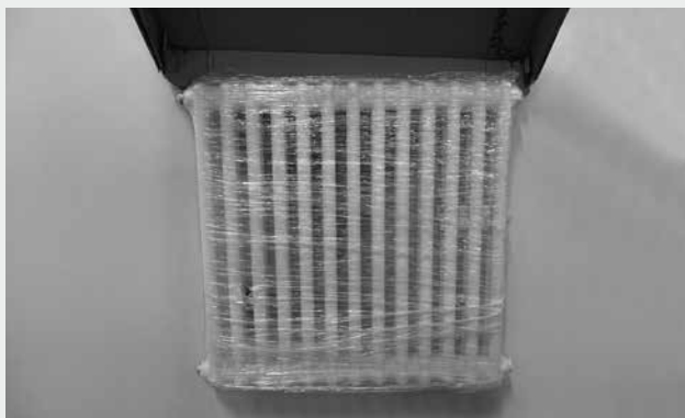
Stretch film remains in place during installation and protects the radiator until you move in.
