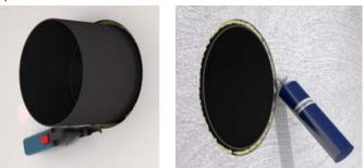
Position the bottom cover of the exterior wall panel centrally on the PVC wall mounting pipe, maintaining a distance of x = 33 mm, and align it horizontally with the façade. Transfer the drill holes and prepare a suitable fastening technique for the four fixing points (shown as long holes) as set out in the façade design.
