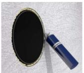
Glue the swelling sealing tape from the ComfoAir 70 accessories to the contour on the back of the exterior wall panel bottom cover.
